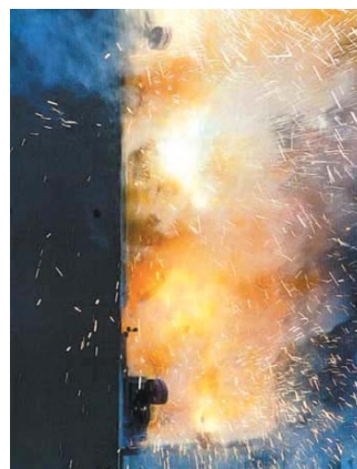
Photograph by Square D/Schneider Electric
