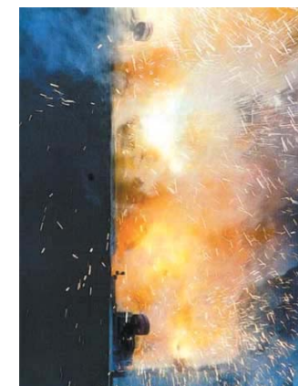
Photograph by Square D/Schneider Electric
