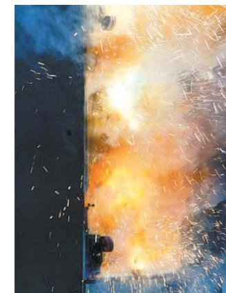
Photograph by Square D/Schneider Electric
